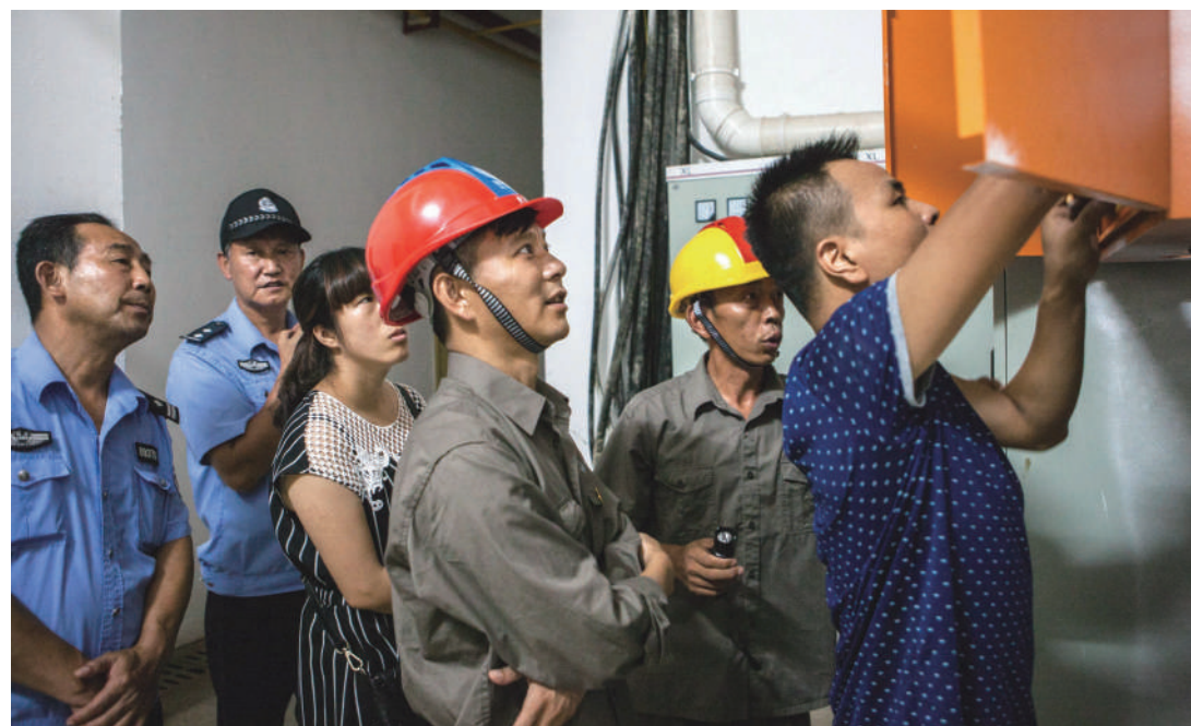
稽查人员在崇尚华府小区检查配电房。邓东峰/摄
